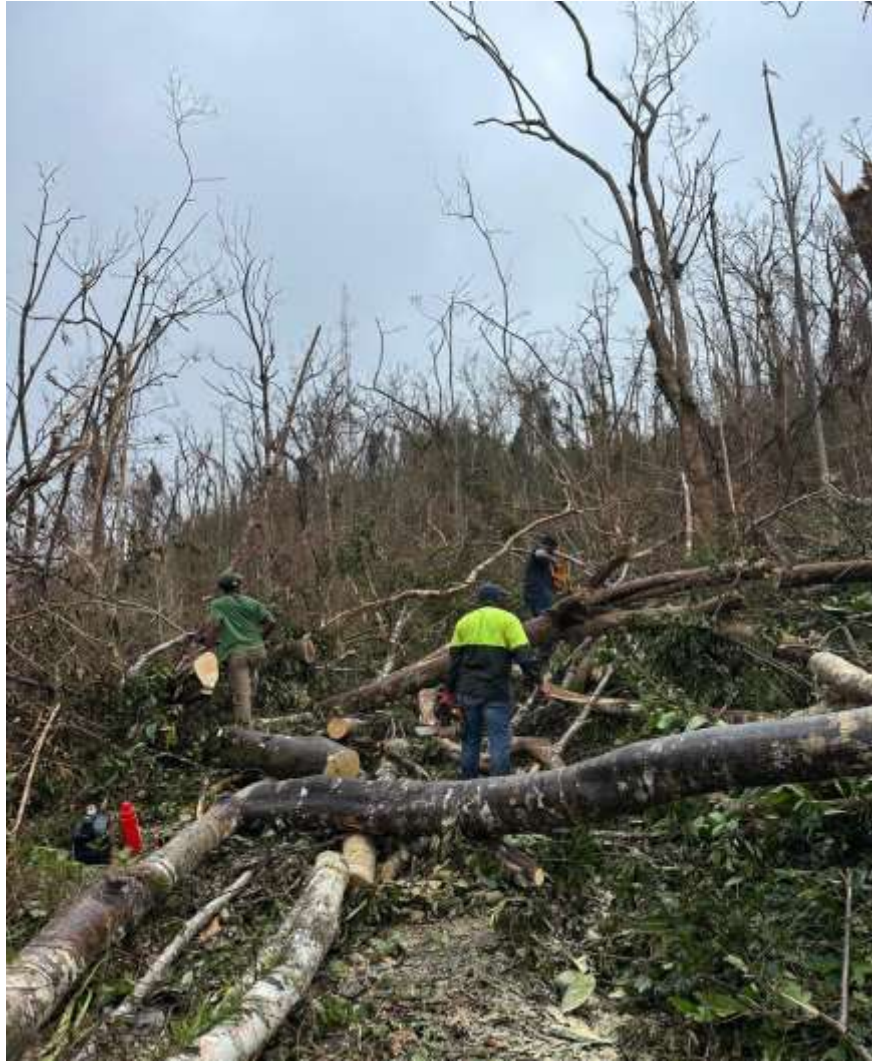
'Clearing' our way on the main road to the site
